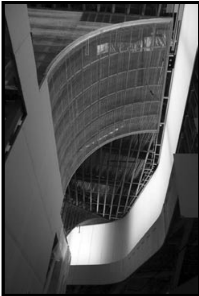
An interior “flutter wall” at the Bloch Building expansion at the Nelson-Atkins Museum. Photo courtesy Nelson-Atkins Museum.
