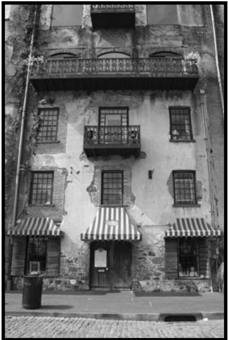
An old building on the Factors' Walk in Savannah, Georgia.
